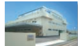
No. 2 Kakamihigashimachi Plant (Gifu Prefecture, Japan)
