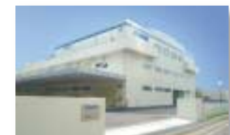
No. 2 Kakamihigashimachi Plant (Gifu Prefecture, Japan)
